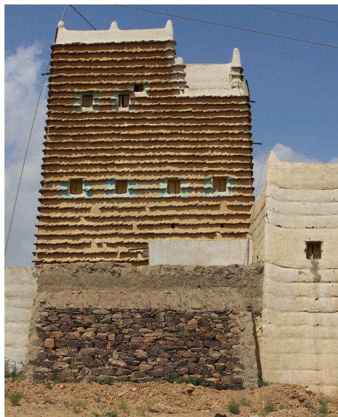
FIG. 25 Vernacular architecture in Ahad Rafidah
