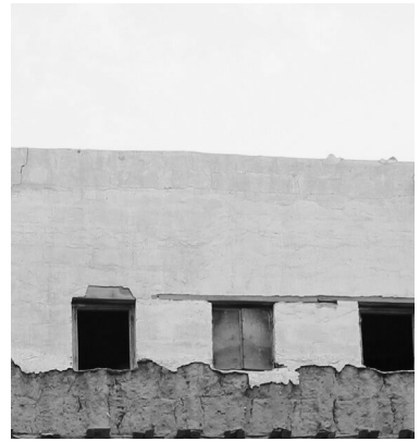
Flat plastered rooftops
