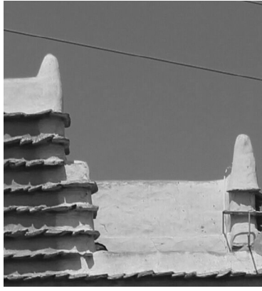
Pointed parapet wall corners
