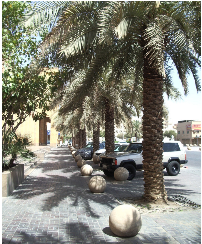
FIG. 70 Vehicular bollards using reconstituted stone and local materials. Qasr Al Hukm, Riyadh, KSA
