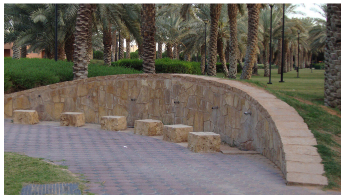
FIG. 71 Retaining boundary walls, and seating elements utilizing local natural stone, Salam park, Riyadh, KSA
